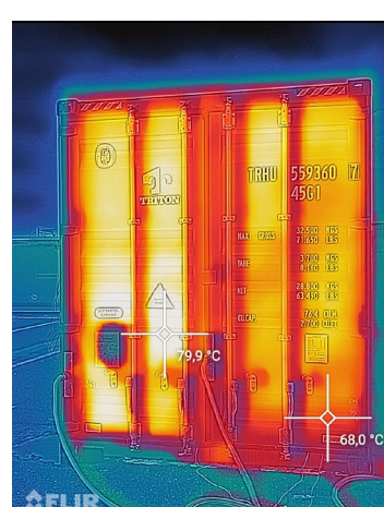
Door area – Infrared thermography identifying the artificial cold-point reference zone generated by the injection methodology
