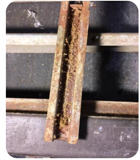
Khapra beetle infestation from underfloor area
