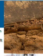
soil under container
