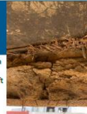
soil under container
