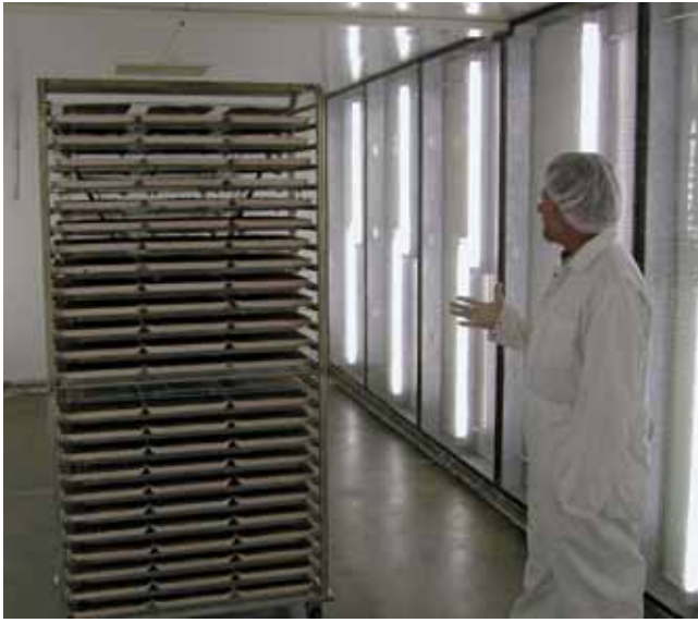
FIGURE 32 Rearing room with vertical fluorescent tubes in the air plenum behind clear-plastic walls – OKSIR mass-rearing facility, Osoyoos, Canada.
